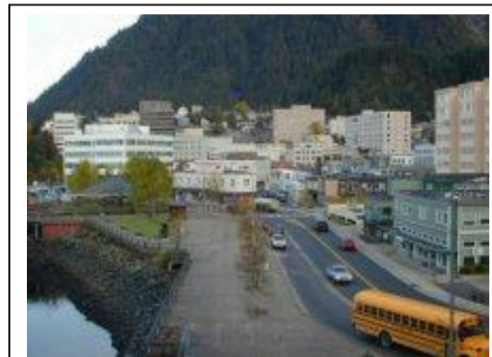
Structures at risk in the high hazard area.
