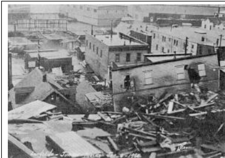
January 2, 1920 landslide damage, looking down from Gastineau Avenue.
