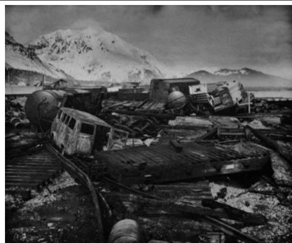
Tsunami damage at Seward, Alaska
