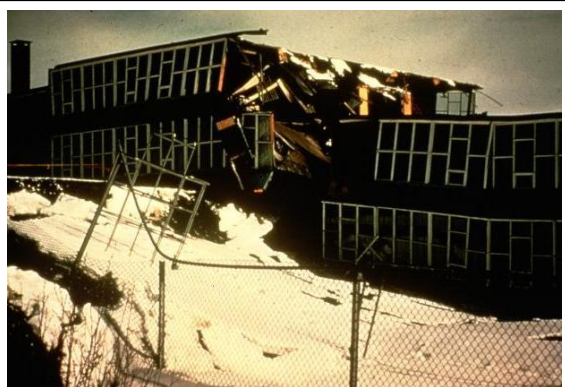
Earthquake damage to buildings in Anchorage, Alaska after the 1964 earthquake.
